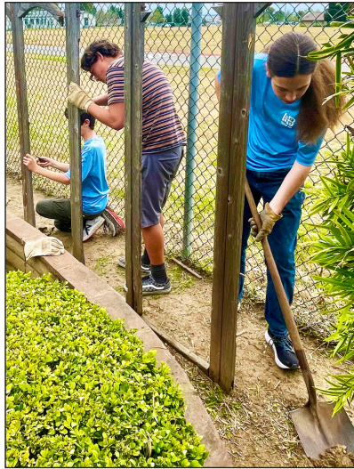
Removal: out comes the old.
